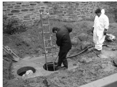
Decon of Tank (removal of mud from shoes)
