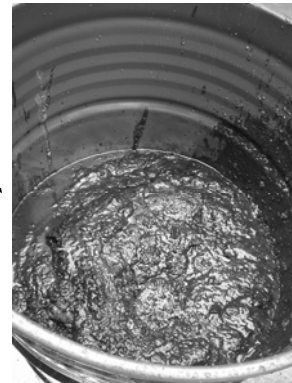
Sludge removed from tank.
